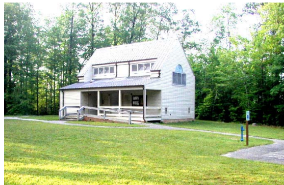
Bath house for E-1 campers, with hot water, private showers, and normal amenities.
