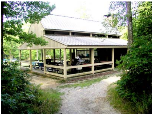
Covered pavilion, with picnic tables and benches and a real fireplace.
